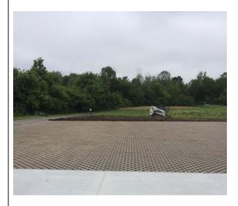
Machine called a Rock Chucker was used to broadcast the topsoil over the grass pavers.
